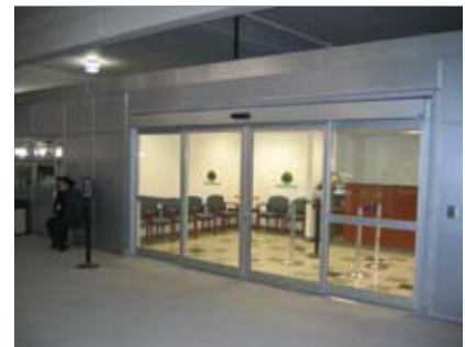
The pre-engineered design of our modular wall systems enabled this car rental agency to construct their new rental office in a fraction of the time required for conventional construction.
