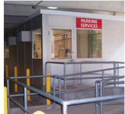
Ballistic rated walls were incorporated into this modular garage office to enhance security for personnel during off-peak hours of operation.
