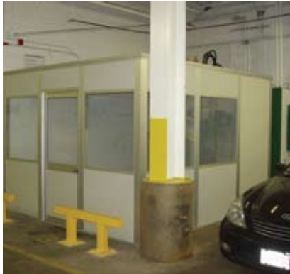
Modular walls were used in this previously used corner of this parking garage to create a clean, comfortable office space for security personnel.
